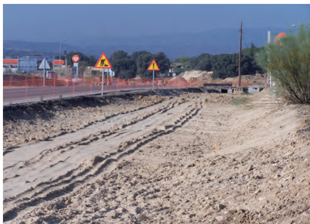
M-501 under construction
